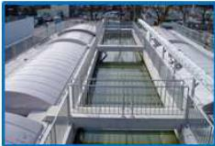
2. HOFFSELVA Local Treatment of Combined Sewer Overflows
