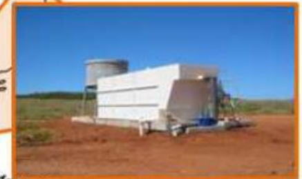
4. ATHENS AMI-Enabled Sewer Mining for water reuse
