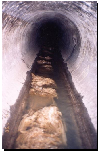
sedimentation and erosion of sewer deposits
